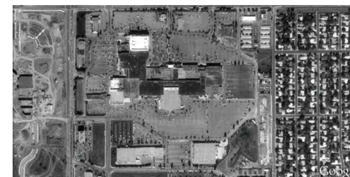
Belmar – Lakewood, CO (old Villa Italia Shopping Mall) new town center mixed-use development
