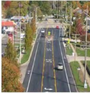
Center turn lanes, bike lanes, and pedestrian refuge island at bus stop
