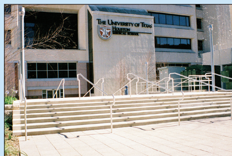
Figure 3-25. Three sets of stairs that provide building egress during the design flood event, but still allow normal use of the building (source: Walter P. Moore)
