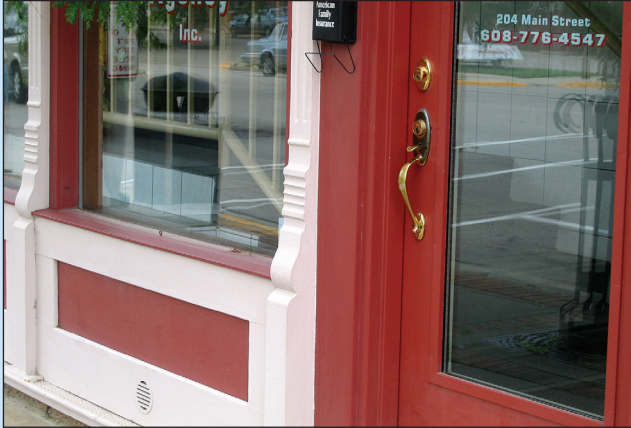
Figure 4-32. Hardware store on Main Street in Darlington, WI, (left) mitigated with a raised interior first floor and flood damage-resistant materials (right)
