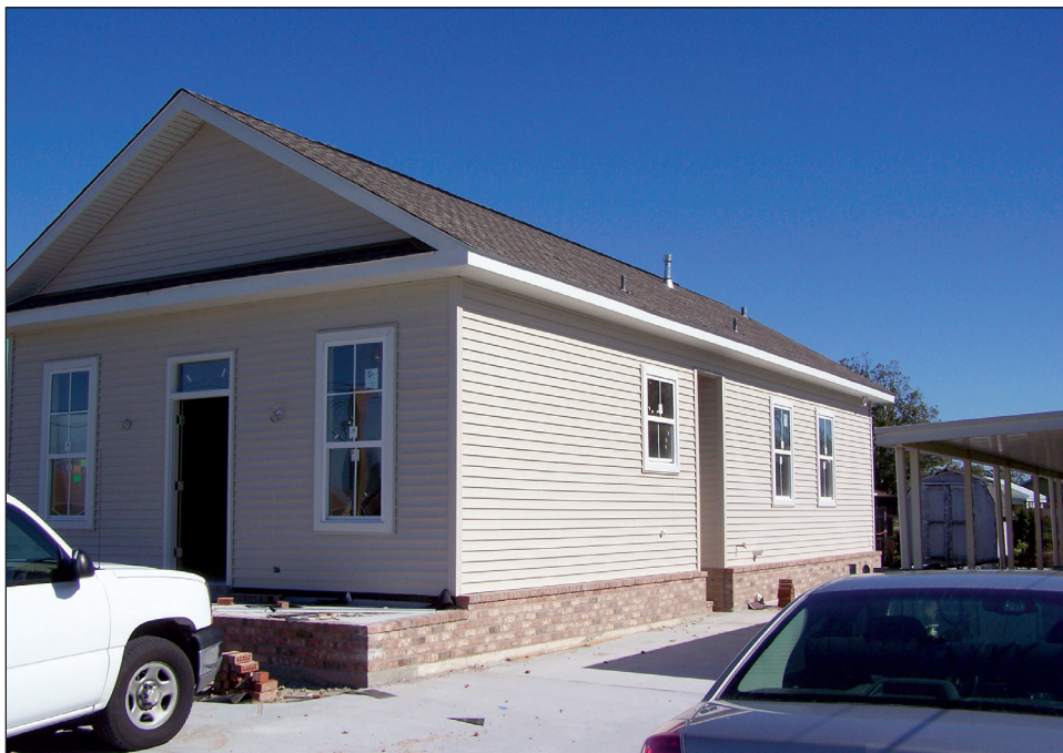
Figure 6-9. Typical mitigation reconstruction project.
