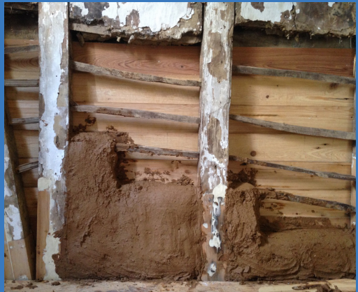
Bousillage infill hung on rungs between posts
