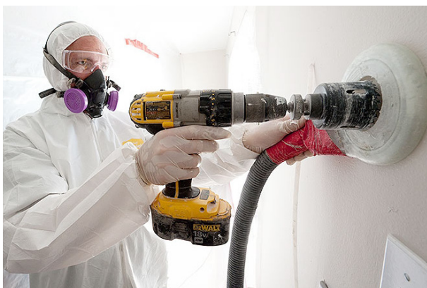
[Source: Energy.gov (photo by Dennis Schroeder). A weatherization worker drills holes to blow cellulose insulation in the interior walls of this home.]
