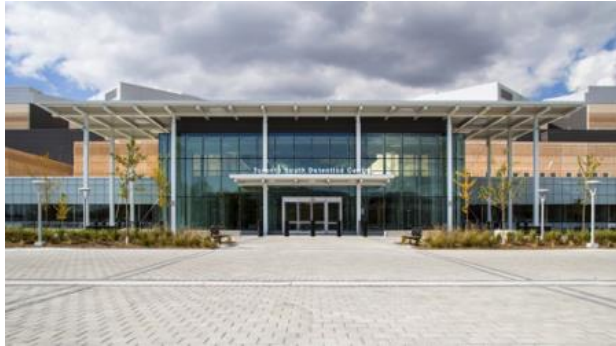
Toronto South Detention Center
