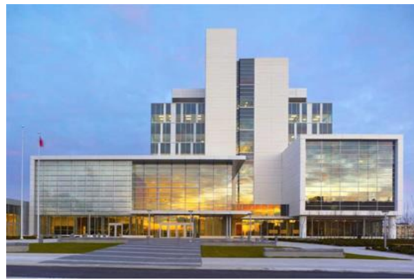
Durham Region Courthouse
