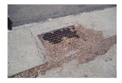
BAD: Grass and leaves blown into a storm drain interfere with drainage. Dirt is also being allowed in our waterways.
