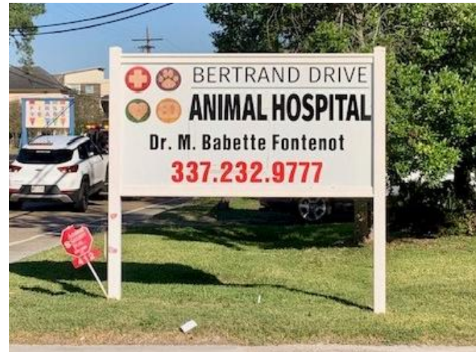
Pole Sign (2 structural poles)
