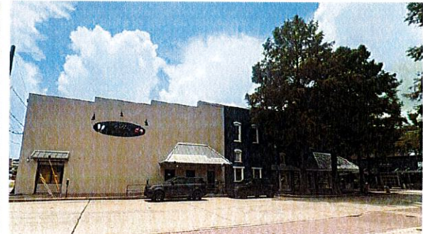
Side / rear condition
